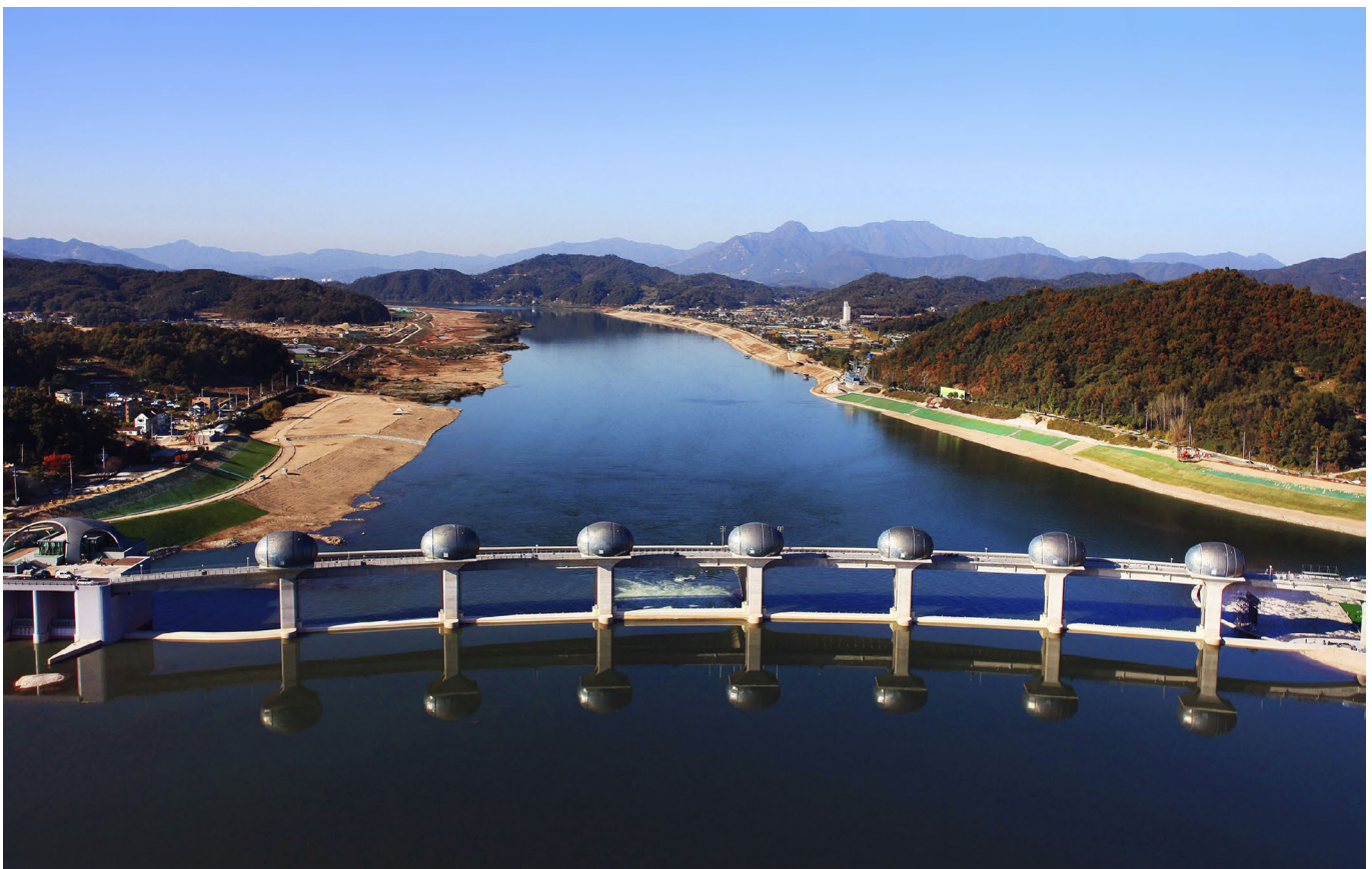
Figure 2 | The curved-shape Ipo Weir across the Hang-gang River (Courtesy of Yeosu City).
